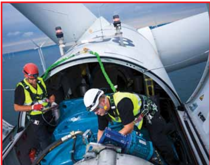
Routine maintenance performed up-tower (courtesy of Siemens)
