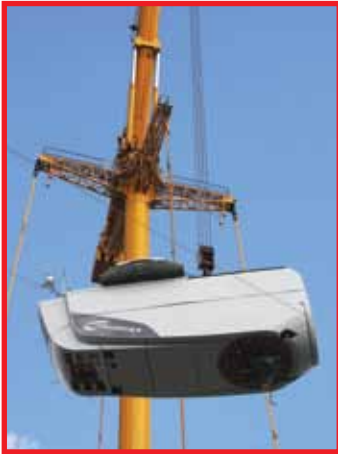
Nacelle housing gearbox and generator being hoisted during installations (courtesy of Nordex)
