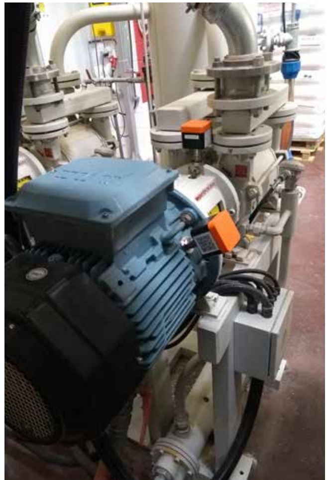
Remote wireless monitoring of the vibration patterns of rotating machinery has revolutionised condition monitoring. The remote sensors (pictured) are 'on duty' 24 hours a day, keeping the machine under constant surveillance while transmitting the data wirelessly, thus reducing the risk of failure.
